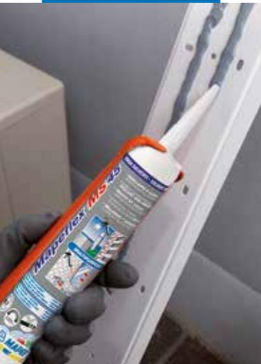
Bonding plastic profiles on a surface outside
